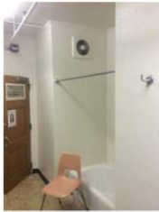
6. TUBS AND VENTING - Vents directly into the janitor closet
