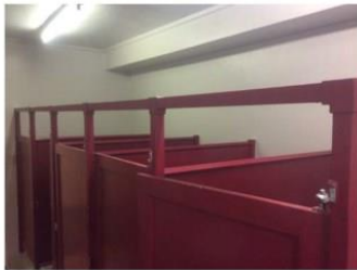
10. TOILET PARTITIONS & LIGHT FIXTURE - Exposed lamp on light fixture
