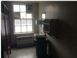
6. WINDOW AND VENTING - Single pane glazing and inappropriate venting
