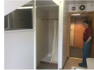
4. LOOK BACK TO ENTRY - Inappropriate venting into the hall
