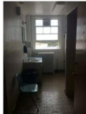
3. BATHROOM SINK - dated fixtures and casework: Not ADA compliant
