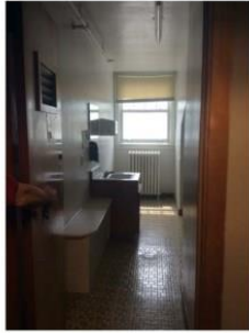
1. FROM BATHROOM ENTRY - Exposed lamp on light fixture; tight space at entry, dated finishes and fixtures
