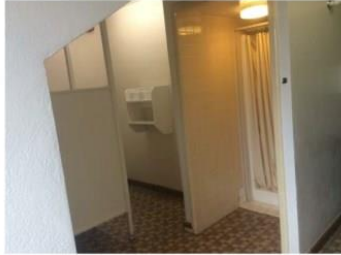
1. SHOWER and TOILETS UNDER SLOPE - May be code non-compliant for ceiling height
