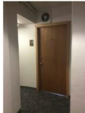
2. ENTRY TO BATHROOM 1 - Inappropriate venting from bathroom
