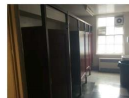
5. TOILET STALLS & LIGHT FIXTURE - Exposed lamp at light fixture
