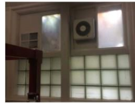
9. WINDOWS AND VENTING - Single pane windows and inappropriate venting
