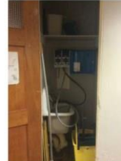
2. JANITOR CLOSET - Small space with narrow door
