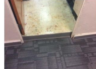
1. BATHROOM FLOOR ELEVATION CHANGE - Trip Hazard, not ADA compliant
