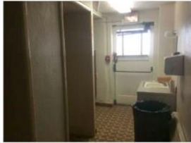
1. FIRE EXIT THROUGH BATHROOM AT 3RD FLOOR
