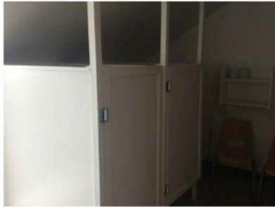
4. TOILET PARTITIONS UNDER SLOPE
