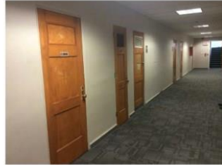
4. CORRIDOR DOORS - Not self closing or fire rated. In appropriate through door venting
