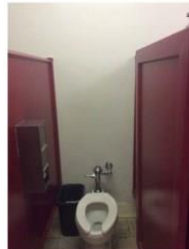
11. TOILET PARTITIONS - Narrow stalls; Lack ADA compliant stall
