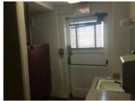
2. FIRE EXIT THROUGH BATHROOM AT 3RD FLOOR
