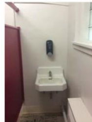
12. SINKS - Narrow sink space; Not ADA compliant
