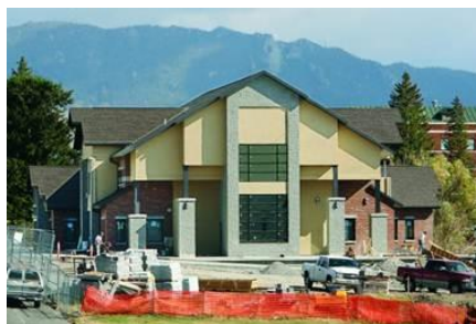
Bike Path Construction at Montana
